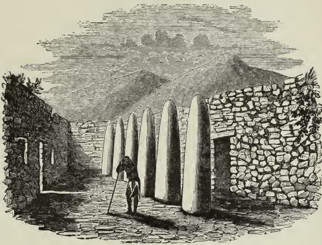
Interior—South wing of the First Palace.
